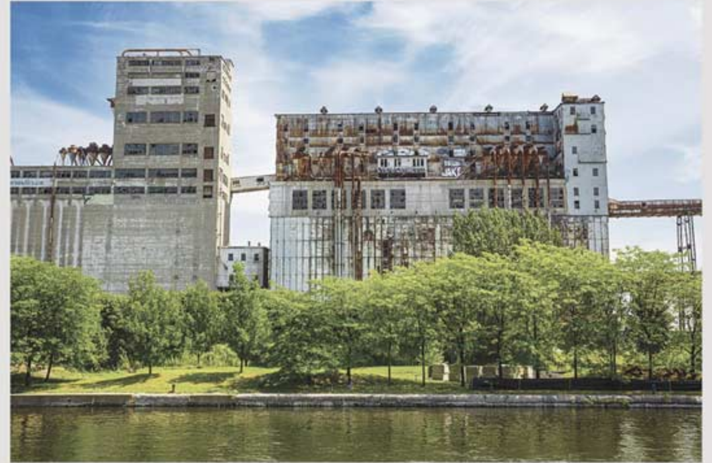
M4- Silo No.5
